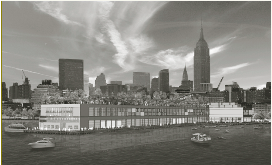
Hudson River Park's Pier 57, as envisioned by Hudson River Park Trust and Youngwoo & Associates. See Profile on page 128. Image: Courtesy of LOT-EK.
