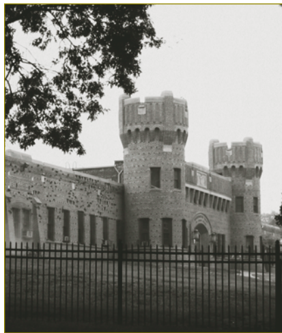
Staten Island Armory in Westerleigh, Staten Island. Image: LPC.
