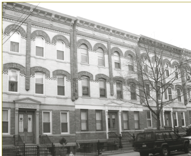
Ridgewood North Historic District. Image: LPC.
