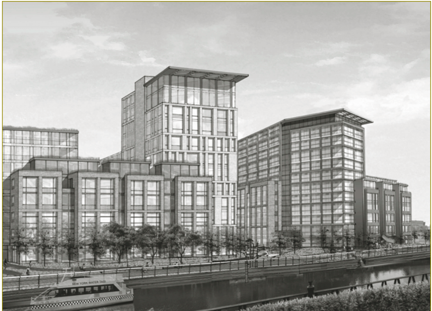
Toll Brothers' proposed development along Gowanus Canal. See story on page 4. Image: GreenbergFarrow.
