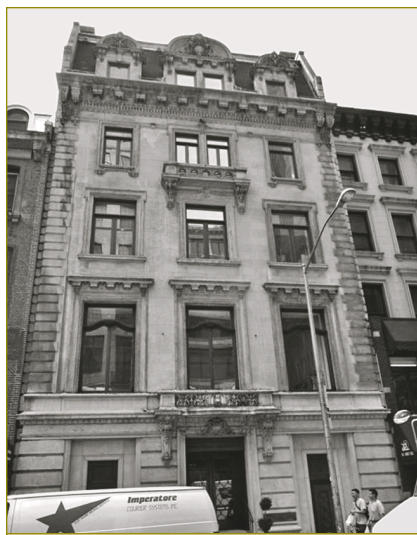
Henry Seligman residence at 30 West 56th Street designated. Photo LPC.
