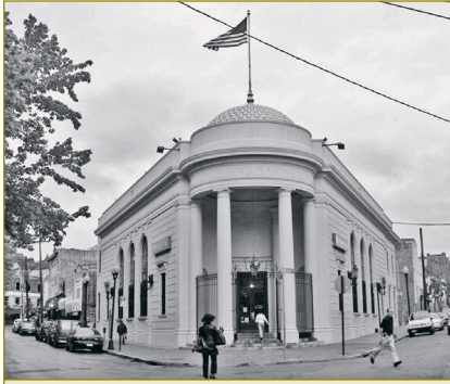
Staten Island Savings Bank designated by Landmarks. Photo: Landmarks Preservation Commission.
