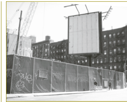
Third Water Tunnel site in Little Italy. Photo: Jeffrey Ocasio.
