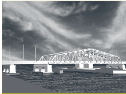
Rendering of the new Willis Avenue Bridge to be built between 125th Street in Manhattan and Bronx's 132nd Street. Used with the permission of the NYC DOT.
