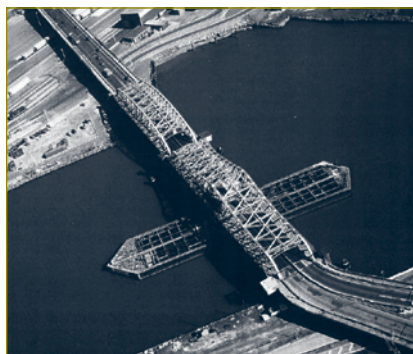
Existing Willis Avenue Bridge at 125th Street to be replaced by DOT. Photo: DOT.
