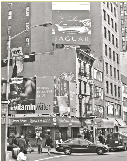
Two-story building in Chelsea to be demolished. Photo: Morgan Kunz.
