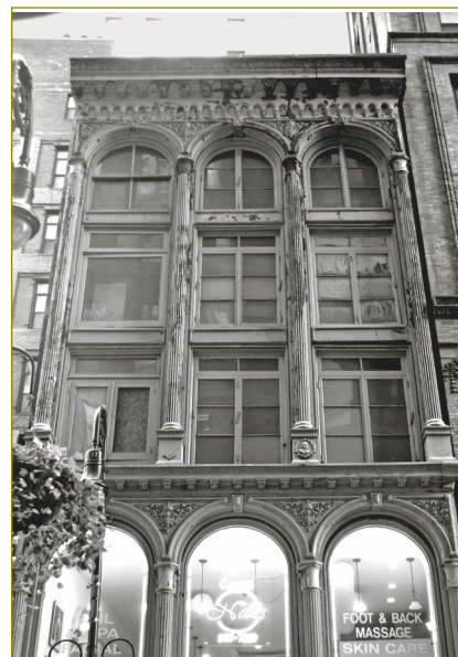
Cast-iron building at 63 Nassau Street considered for designation. Photo: LPC.
